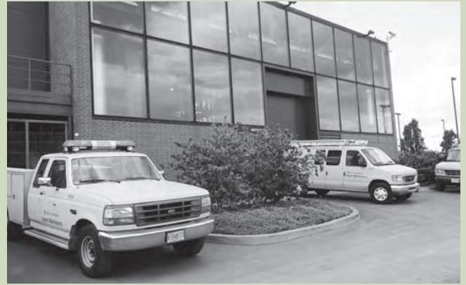
The upgraded Central Utility Plant at the airport
