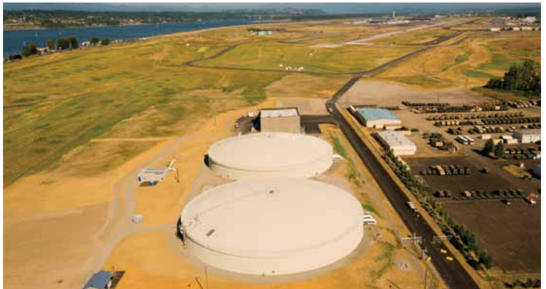
A number of large multi-year Port projects were completed in FY 2010-11. They include the extension of the north runway, the baggage screening improvement project, and airfield deicing system enhancements (shown above), at PDX as well as the completion of the Columbia River channel deepening.
